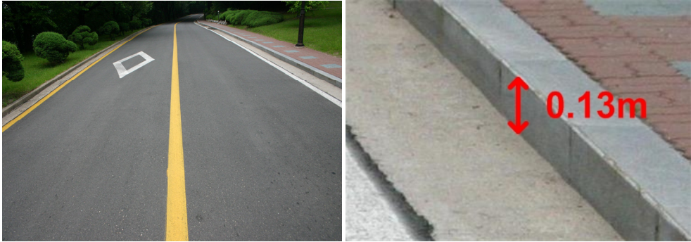
Fig. 3. Road and curb on the road.
