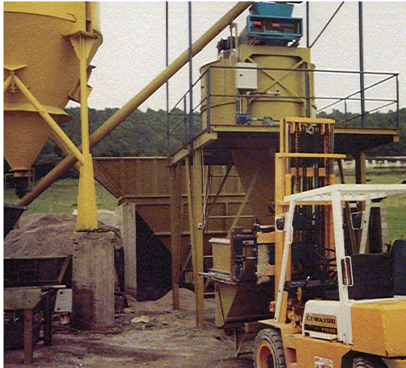
Fig. 5. The materials feeding and mixing platform
