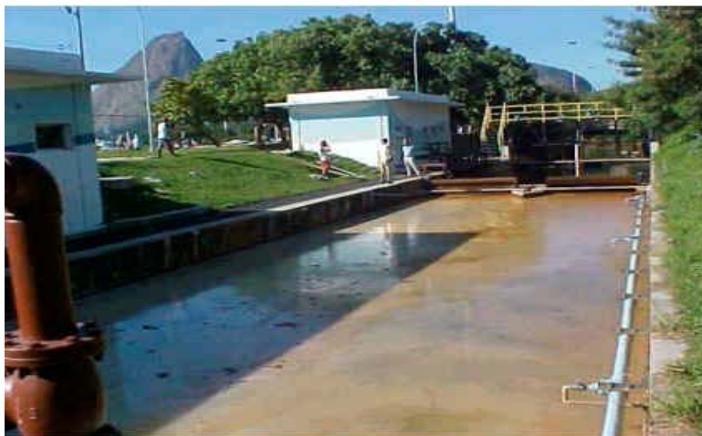
Fig. 4. Treatment station of Flamengo Beach
