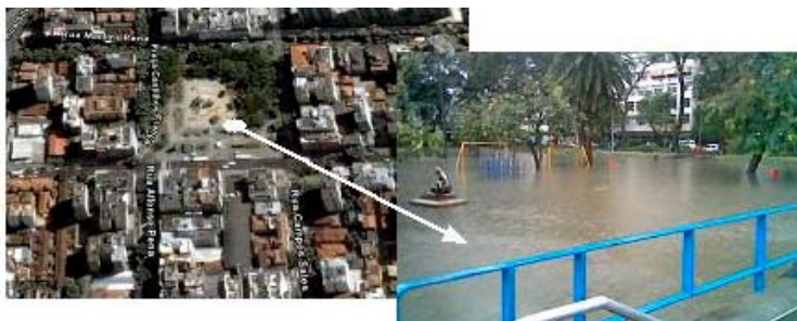
Fig. 5. Afonso Pena Square, acting non-intentionally as a detention pond – RJ/Brazil
