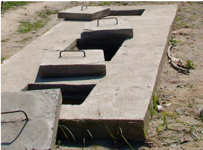
Fig. 7. Photo of the Guerengue road sand filter
