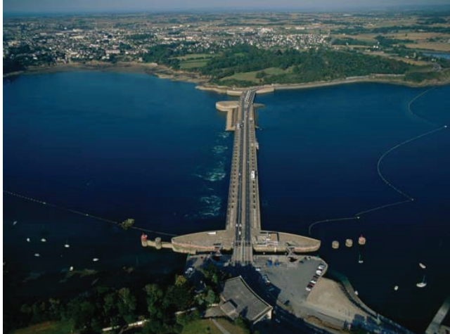
Fig. 5. Barrage tidal power plant on Rance River (Source: http://www.britannica.com/EBchecked/topic-art/595132/118418/Tidal-power-generation-station-on-the-Rance-River-in-Saint )
