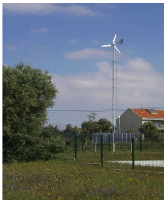
Fig. 2. Wind Generator and PV array of RenH 2 project
